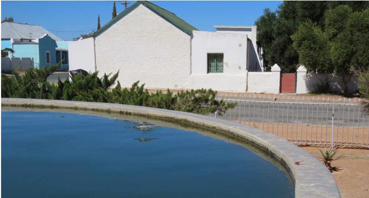
Figure 9: This circular reservoir is in the northeastern corner of the grounds of the Dutch Reformed Church in Vanrhynsdorp. It is a good place to see Orange-winged Dropwing (Figure 10), and occasionally Nomads are seen here too. The males of these two dragonfly species are red, and this is a good place to see them close up, and learn to identify them.
