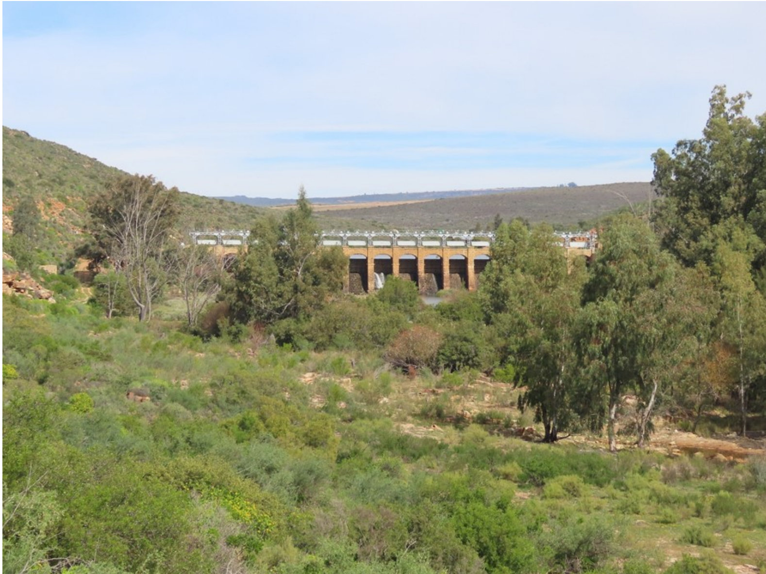
Figure 2: Bulshoek Dam was constructed in 1923 (Box 3). Although the flow of the river below the dam has been dramatically altered, the watercourse and banks are little changed. Thus this section of the Olifants River from the dam downstream to Trawal might be particularly interesting to explore for dragonflies and damselflies. They will be almost absent from the sections where Eucalyptus trees overshadow the river. The year 2023 marks the 100th anniversary of the construction of the dam. There is no public access to this section of the river, and permission from landowners is essential.
