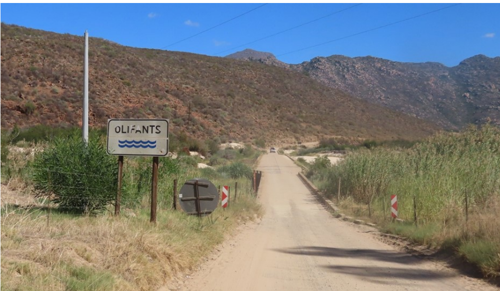
Figure 5: The Algeria bridge. This low level bridge is roughly halfway between Citrusdal and Clanwilliam, 2 km from the N7 along the road that leads to Algeria Campsite in the Cederberg (Figure 1). Bridges like this provide good opportunities for seeing dragonflies and damselflies.
