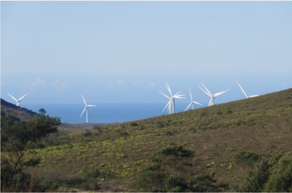
Figure 2: Wind turbines at one of the operational windfarms.
