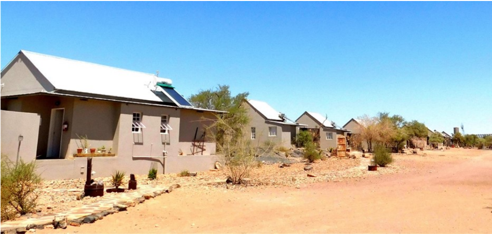
Figure 14: Alte Kalköfen Lodge offers an array of accommodation options: chalets, self-catering cottages and camping. The building on the left is one of the two self-catering cottages; with some of the 10 chalets beyond it. The camping site is about 100 m to the right of this photograph.
