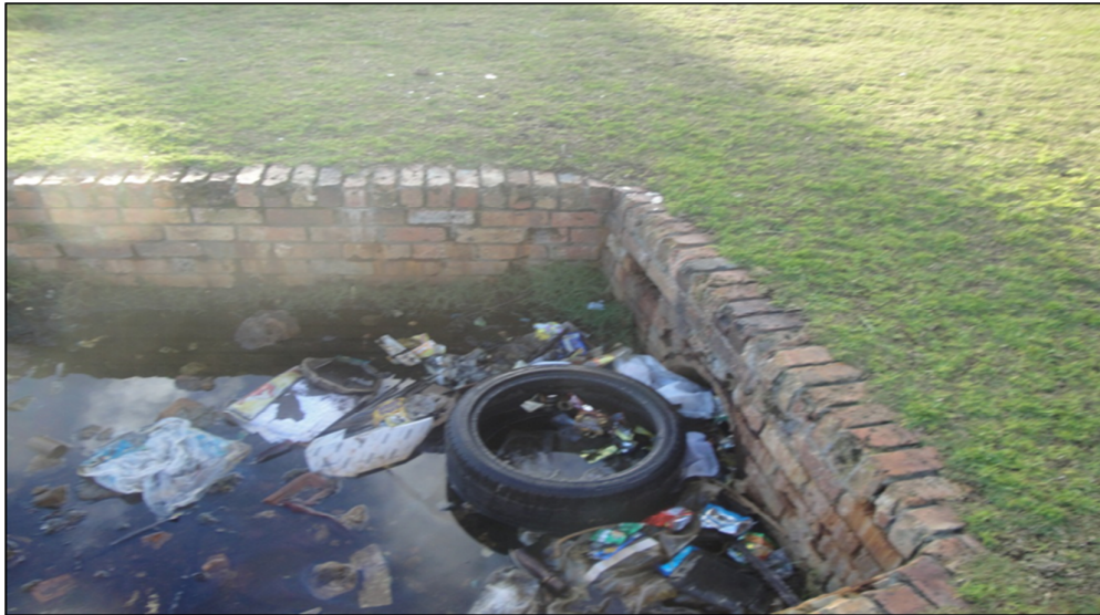
Figure 6: A stormwater pond classified as 'litter trap' due to litter accumulating in the outlet
