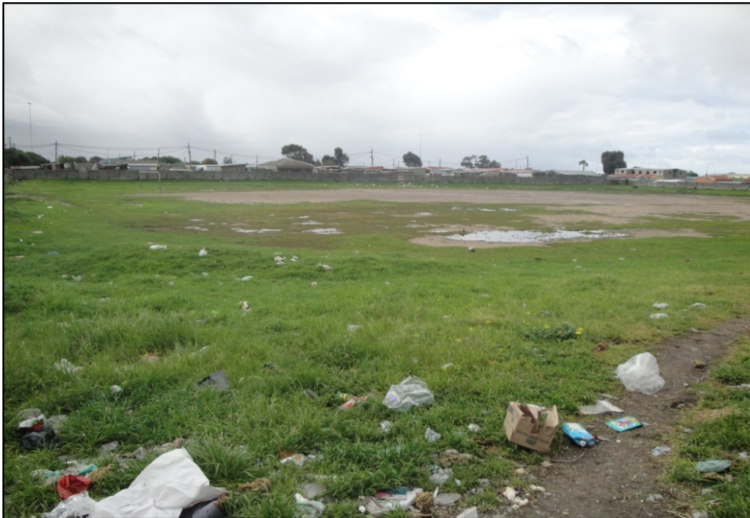
Figure 3: A detention pond in a low affluent area in which dual use has led to the erosion surface material
