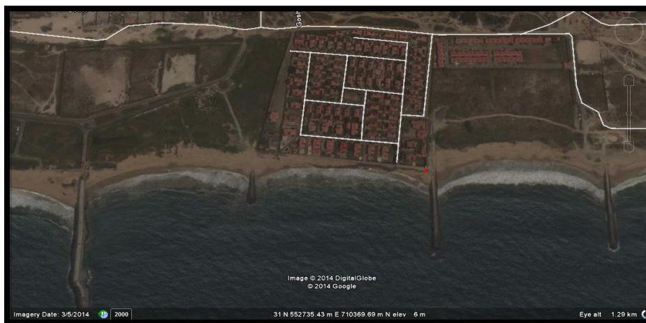
Plate 3.2. Google imagery of 5/3/2014 showing newly constructed groins around Goshen Estate and new u-shaped erosion/accretion between the groins. The new groins are apparent confirmation of extant serious erosion.
