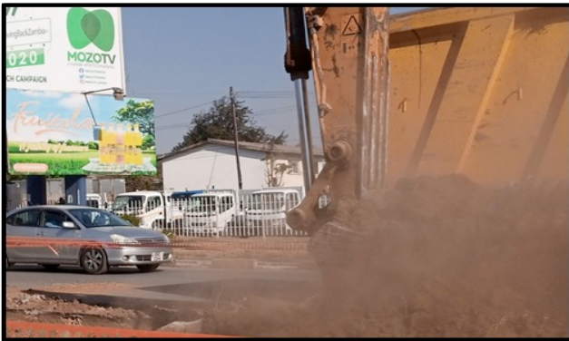
Figure 3: Picture depicting dust exposure during loading of spoil
