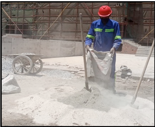
Figure 7: Picture showing cement dust exposure during dry mixing
