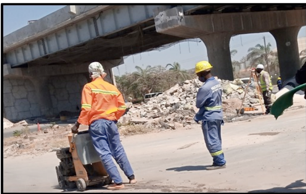
Figure 10: Picture showing the use of a cutter with water on the road project
