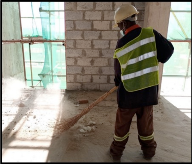
Figure 6: Picture showing dust exposure during dry sweeping
