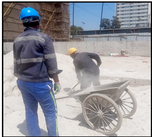
Figure 5: Picture showing workers loading quarry dust for batching
