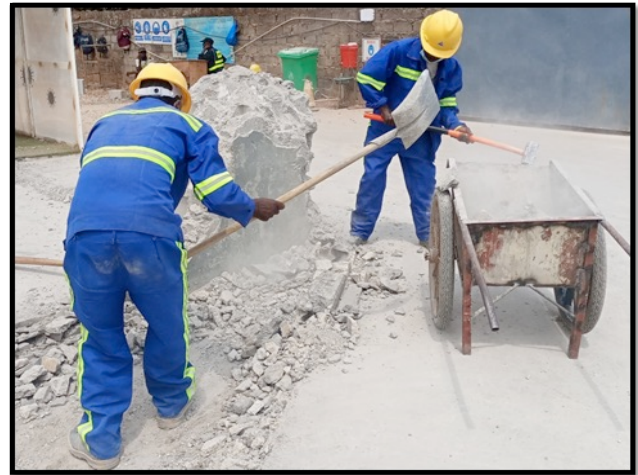
Figure 8: Picture showing dust exposure during demolition and loading of rubble
