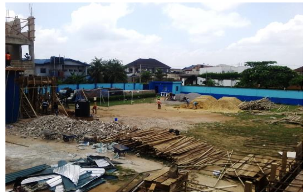
Figure 3: Workers at work on construction site (Kukoyi and Smallwood, 2016)
