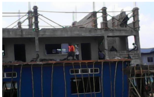
Figure 4: Workers at work on construction site (Kukoyi and Smallwood, 2016)
