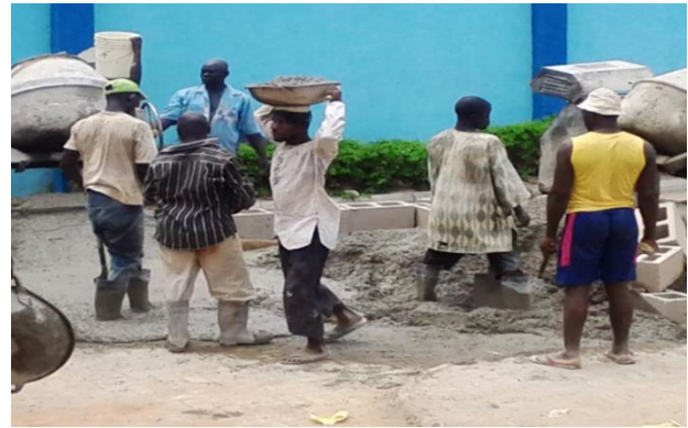
Figure 2: Workers at work on construction site (Kukoyi and Smallwood, 2016)
