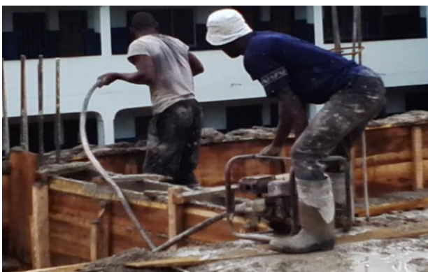
Figure 1: Workers at work on construction site (Kukoyi and Smallwood, 2016)
