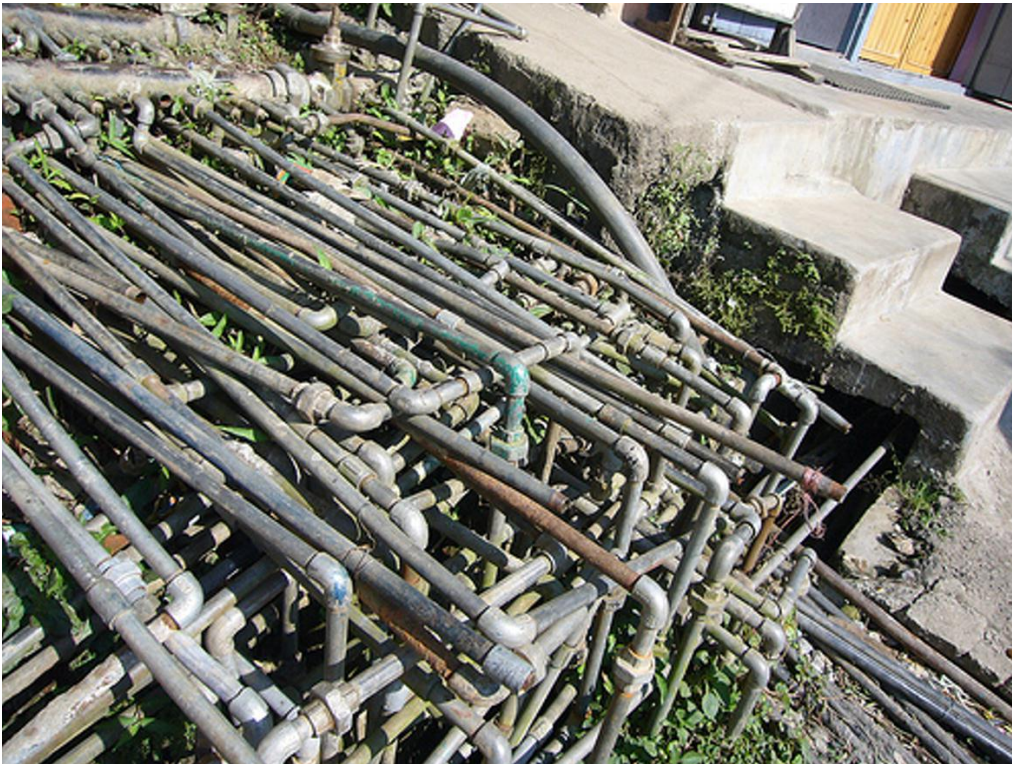
Figure 2: Urban water connections: some may be illegal. Hyderabad 2009 (Domal, 2010)
